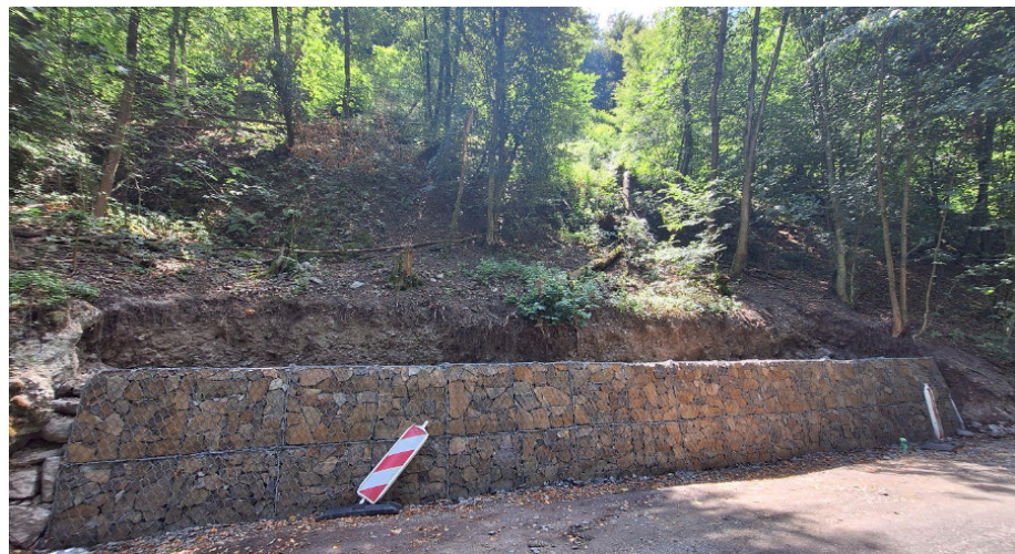
Figure 4. Ongoing gabion construction at the DEMO4 Pusty hrad slopes locality.
