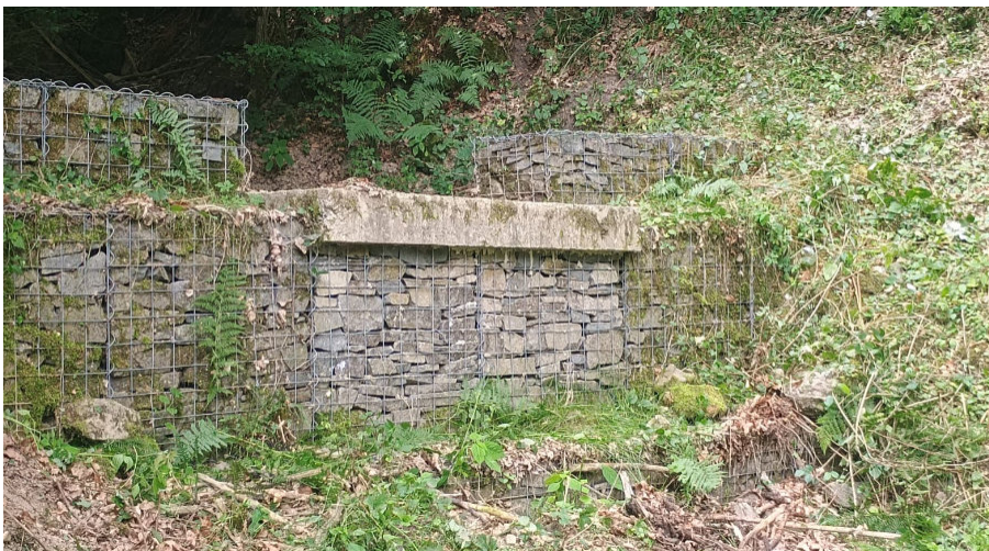
Figure 5. Cleared check dams at the DEMO4 Neresnica locality.
