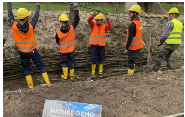
Figure 5. Implementation of a wattle fence.
