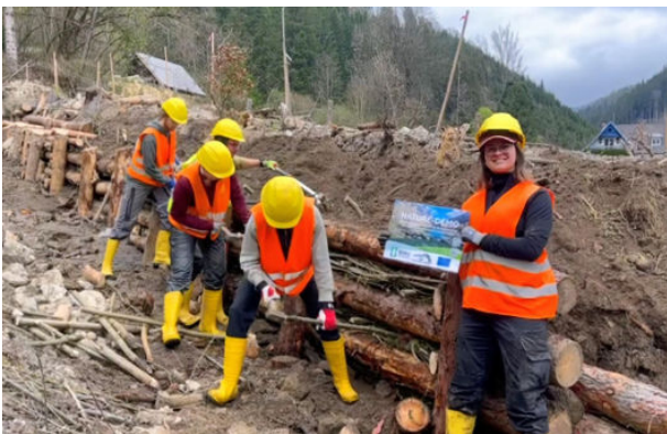
Figure 4. Implementation of a live cribwall with live stakes being merrily hammered in and around
