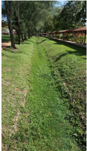
Constructed Swale in USM Engineering Campus
