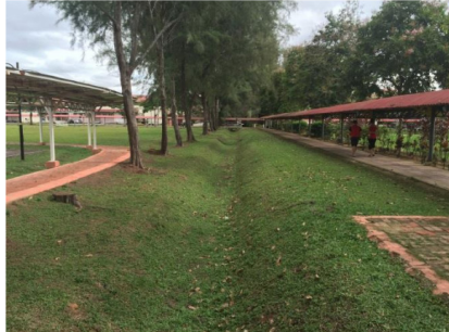
Constructed Swale in USM Engineering Campus
