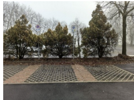
Permeable pavement in Milan, Example of installation (IRIDRA, 2024)
