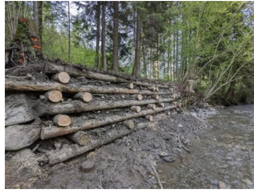
Live cribwall after construction at Veitschbach
