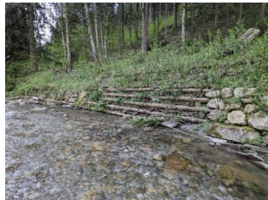
Live cribwall two years after construction at Veitschbach
