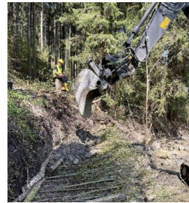
Covering of layer construction with slope sediment, Veitschbach, Styria;
