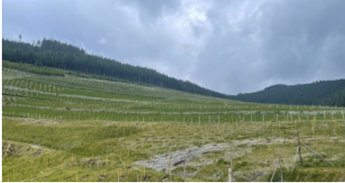
Large scale net greening with biodegradable coconut fibres and subsequent afforestation; Fröschnitzgraben, Lower Austria (A), 2024. Image Credit: [Rosemarie Stangl], [2024], Used with permission
