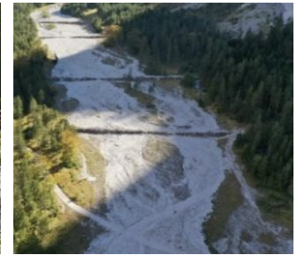
2. Consecutive wooden log fences in a river bed retaining and stabilising large quantities of sediment (Demo-Site Brunnsee)
