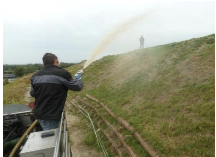
Hydroseeding application as overseeding and for greening bare spots in Vienna Image Credit: [Michael Obriejetan, archive BOKU-IBLB], [2014]. Used with permission
