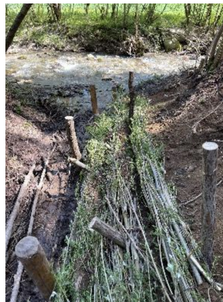
Live fascine row under construction, Veitschbach, Styria (A);
