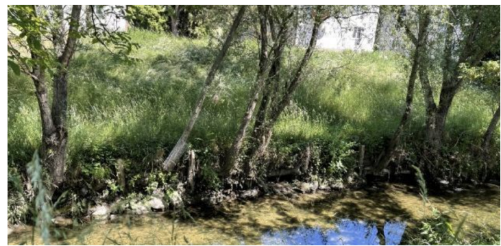
Trees growing from a fascine wall 20 years after installation, Liesingbach (A);
