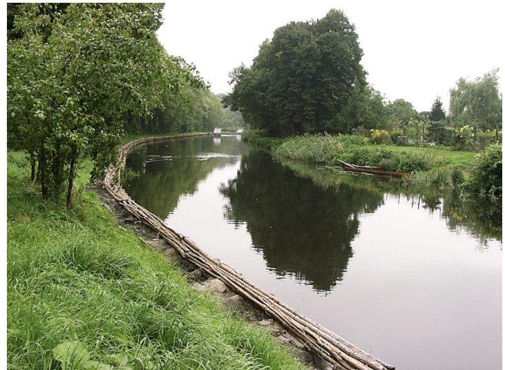
Live fascines at riverbank in Templin, Germany - implementation process, earth substrate to be incorporated on top for triggering budding without suppressing shoot growth Image Credit: [Sebastian Wallroth], [2006], Public domain.
