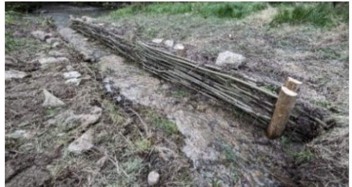
Wattle fence at Veitschbach, Styria (Austria); Image Credit: [Tina Vorstandlechner], [2024]. Used with permission;
