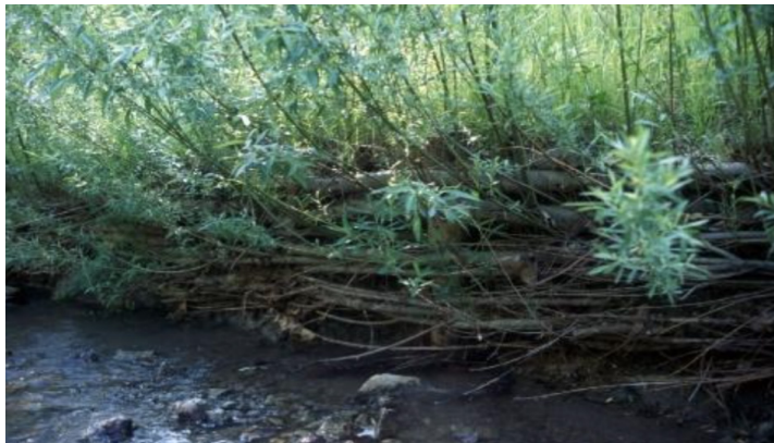
Detail of wattle fence two years after installation, Alsbach Vienna (Austria); Image Credit: [Florin Florineth, BOKU-IBLB archive], [1995]. Used with permission;
