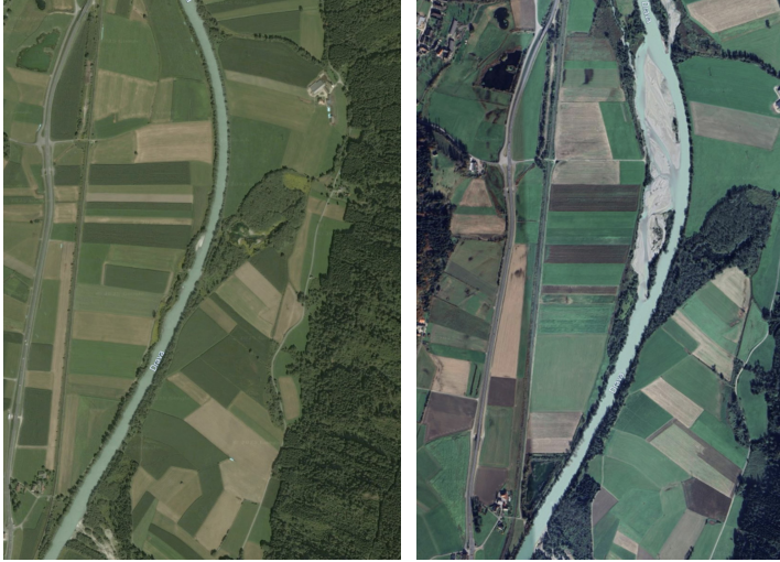
River Drau at Obersgottesfeld (Austria) before (2003) and after (2024) restoration works and channel widening.
