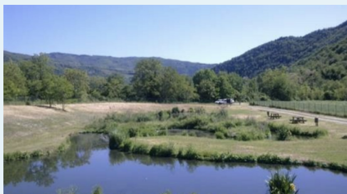
Constructed wetland for wastewater treatment of the City of Dicomano (FI) Image Credit: [IRIDRA], [2003], Used with permission.
