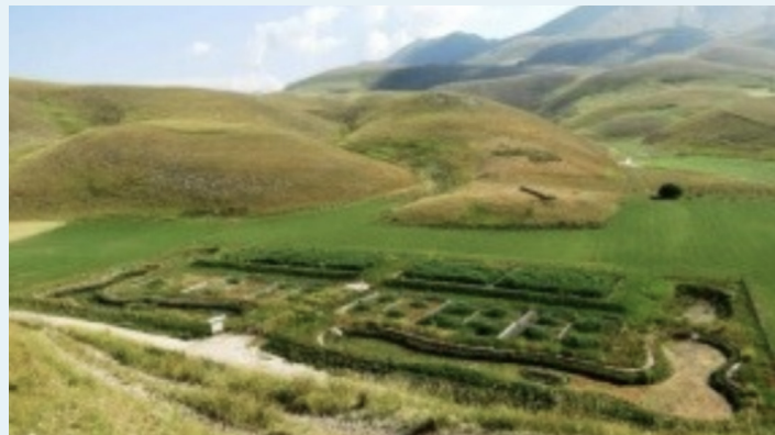
Constructed wetland for wastewater treatment of the City of Orheit (Moldova) Image Credit: [IRIDRA], [2012], Used with permission.
