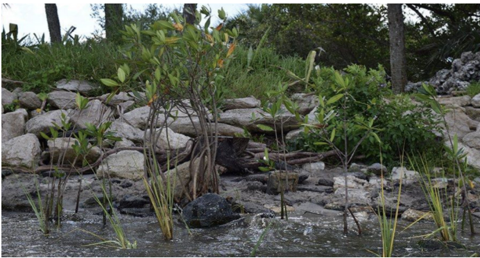
Right: Oyster bag revetment at Douglas Park seawall
