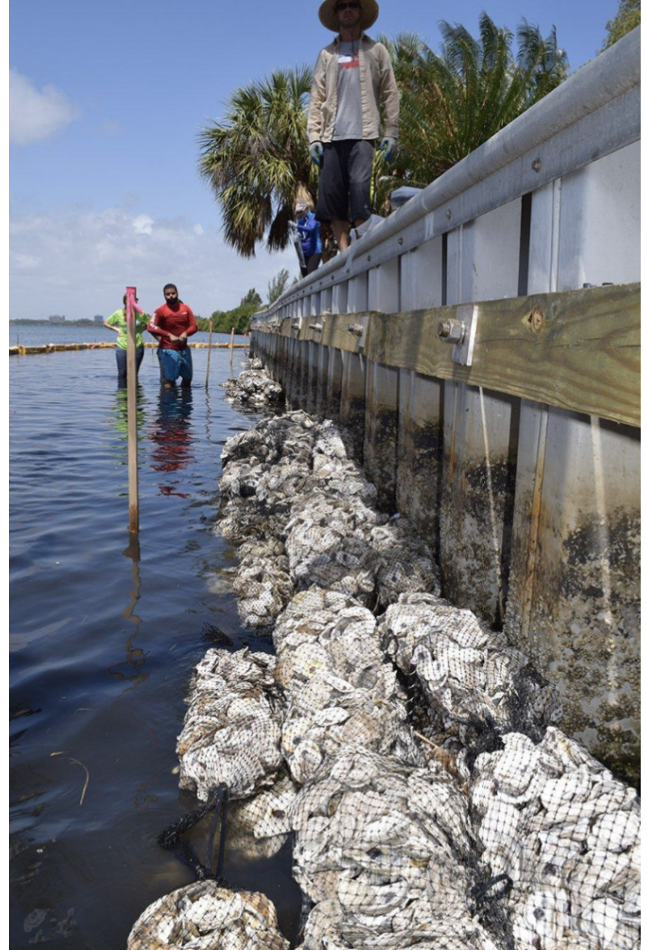
Right: Oyster bag revetment at Douglas Park seawall
